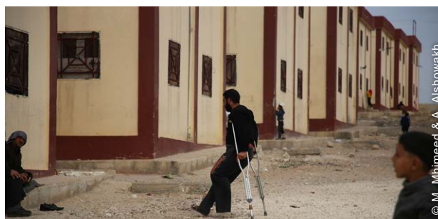
Accessibility was noted as a weakness of the project, with ground floor entrances creating a challenge for people with reduced mobility.
