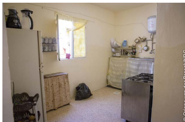
One priority for renovations was to ensure separation of kitchen and bathroom spaces. Here a new wall has been installed to separate the two rooms.
