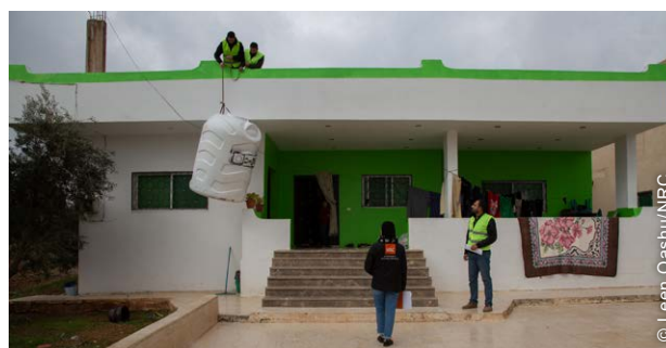
WASH rehabilitation conducted as part of the program, included the installation of water tanks.
