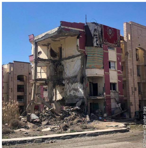
The Shelter Cluster is coordinating with stabilization and development actors on housing rehabilitation/reconstruction, with development actors focusing primarily on urban centers.
