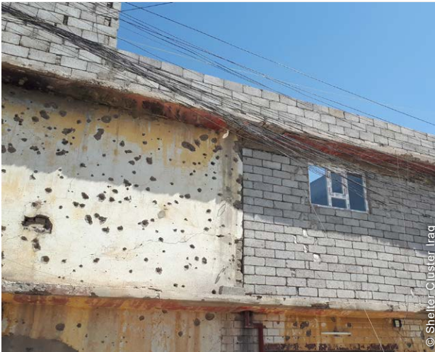
Since the end of the conflict, damage and destruction of housing is one of the key barriers to displaced people being able to return.
