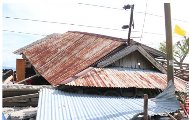
The project involved multiple components, including rubble removal support to help with the clearing of family plots.
