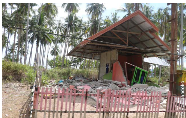
Following the earthquake, 90-95% of homes in Lombonga were severely damaged or completely destroyed.
