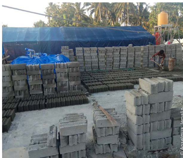
The project engaged local suppliers as much as possible for the production of materials that could be made locally, such as concrete blocks, doors and windows.
