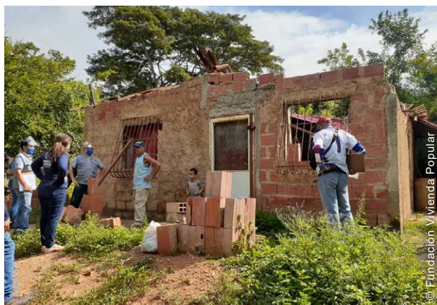
Before and after: housing rehabilitations supported durable solutions for returnees.
