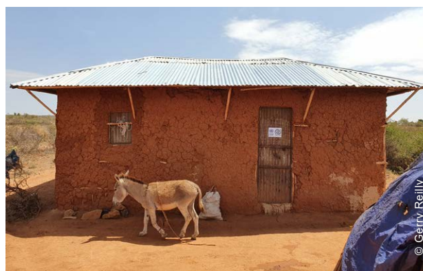
The project supported both households who could repair their partially damaged homes, and households whose homes were beyond repair and needed to be rebuilt.
