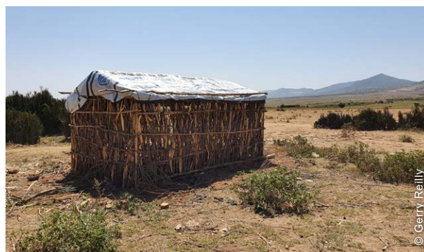
Plastic sheeting distributed in the first installment was used as a temporary roofing material prior to households receiving the second installment.
