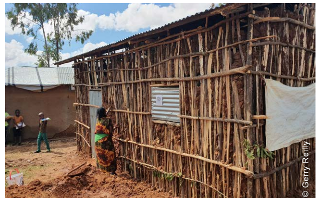
The main shelter typology in East Hararghe is typically a wooden structure that consists of wooden poles harvested locally, wooden infill from wild bushes, and mud plastered walls.
