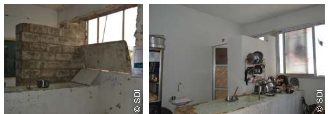
Rehabilitation works included furnishing and upgrade of common kitchens.
