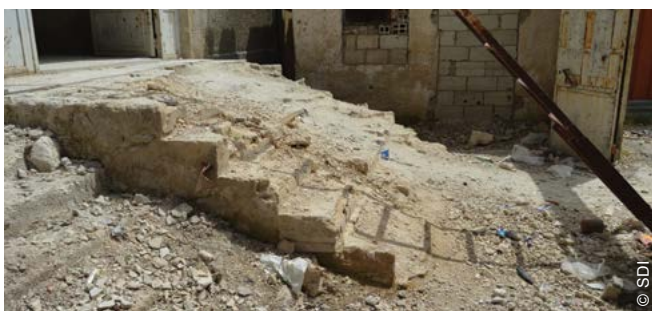
Before (above) and after (right) rehabilitation works in one collective centre.
