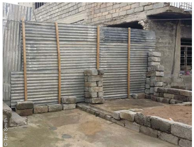
To repair damage to houses, multiple small suppliers were engaged.
