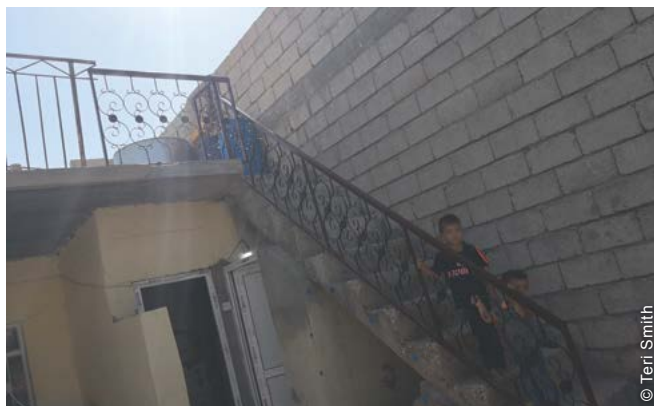
The project repaired walls and stairs, and added handrails for safety.
