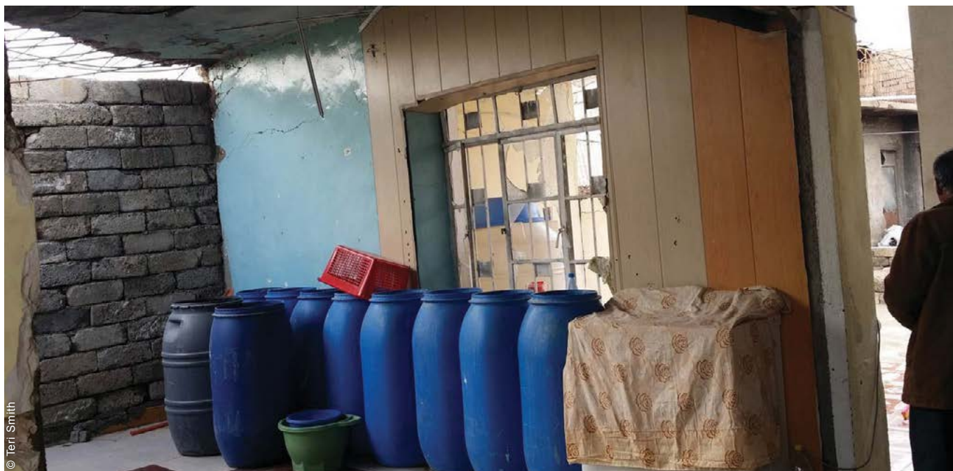
The shelter component of the project focused on repairs to houses in category 1, 2 and 3. This was part of a wider programme including the distribution of household items and the rehabilitation of water and sanitation infrastructure.
