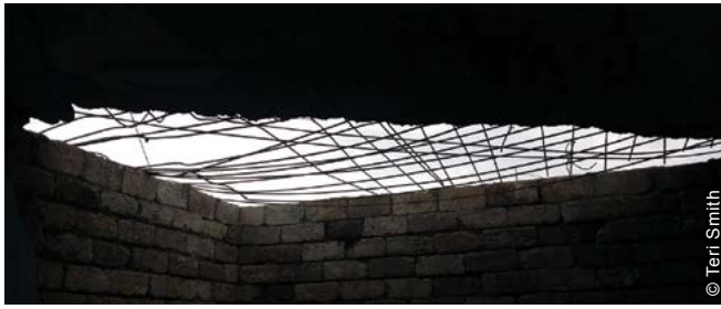
The project rehabilitated houses through a voucher scheme. Repairs included roofs and walls.
