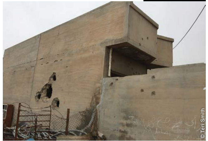
Ninewa governorate was the most affected in terms of displacement and damage to housing.
