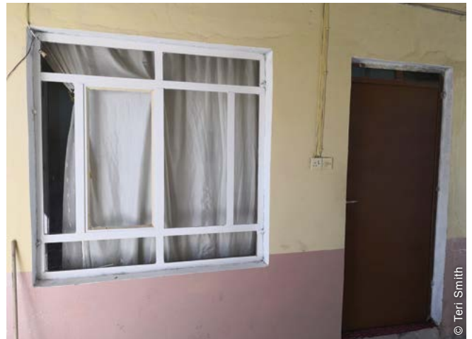
The project also targeted houses with minor damage to avoid tensions within communities. However, this meant that less resources were available for heavier repairs.
