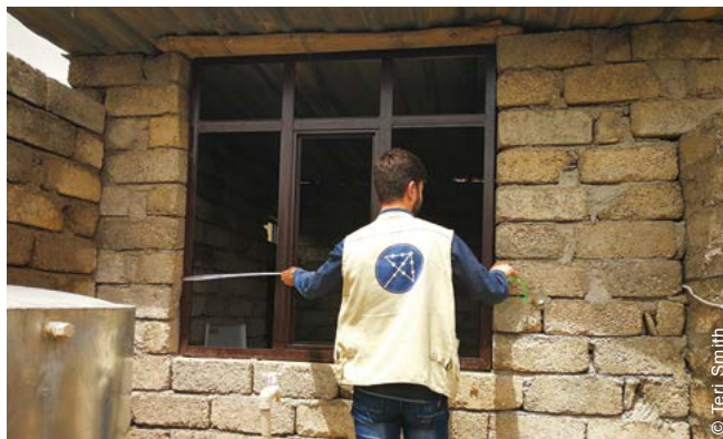
Engineers conducted structural assessments and developed individual BoQs.
