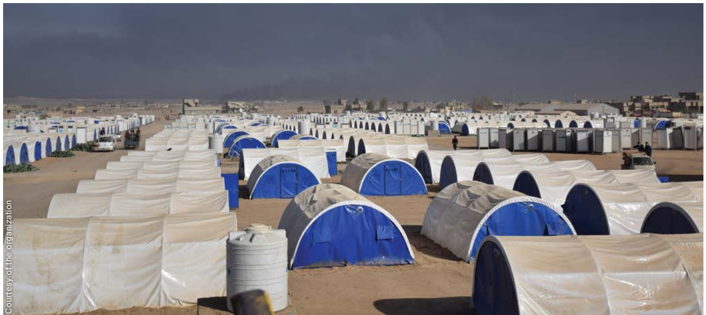
Government standard tents of 6x4m were installed in clustered blocks of 20 each. Space for extensions was minimal but, after families had moved in, upgrades were conducted to the floor and electricity was installed. Partners could then build service facilities in specific blocks pre-allocated in the site plan.
