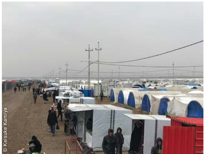
In less than six months, capacity for 17,500 households was established in two sites. The main roads were used for small shops and storage of materials.
