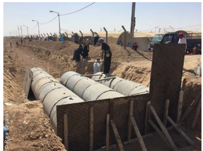
One site was vulnerable to heavy rains and suffered minor flooding during winter. In 2018, storm-water drainage channels and culverts were upgraded.
