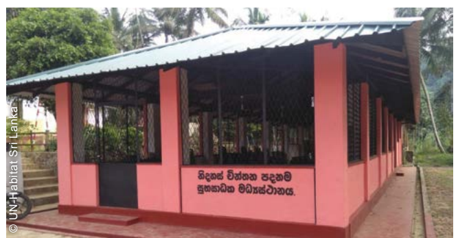
People displaced by the floods found shelter in public buildings. The project upgraded such evacuation centres in cases where families could not go back quickly.
