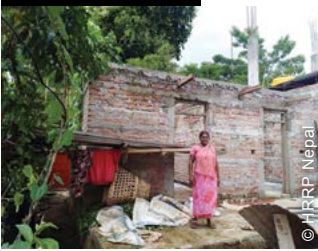
Government grants were used to rebuild a variety of different housing typologies. From load bearing brick masonry and reinforced concrete (above-left) to timber frame and stone masonry (above-right).
