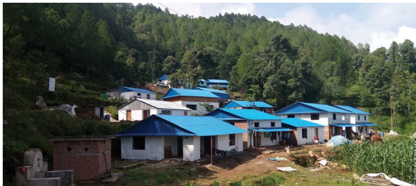
The project provided a holistic support package including shelter, WASH and settlement-wide interventions. It was implemented in close coordination with a variety of government and non-governmental agencies at the national, subnational and field level.
