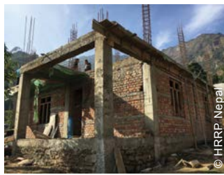
Government grants were used to rebuild a variety of different housing typologies. From load bearing brick masonry and reinforced concrete (above-left) to timber frame and stone masonry (above-right).
