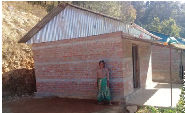
Door-to-door technical support was provided to households, who were divided into groups of ten to support each other during the construction process.
