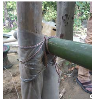
Left (4-5): Cut the required length of floor and roof posts with saw, tie them together and wrap them with polythene sheet. Cut the upper ends of the posts with a fish-mouth cut. Right (6-7): Place and tie floor beams to the bamboo floor post with rope. Place the next set of beams on top, perpendicular to the beam below. Place split bamboo joists above the floor beams. (Photo credits: Habitat Nepal).
