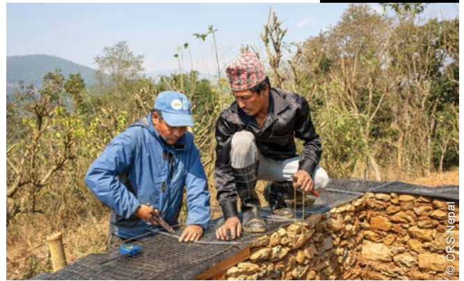
International partners were asked to focus on socio-technical assistance, to support households in rebuilding using earthquake resilient techniques
