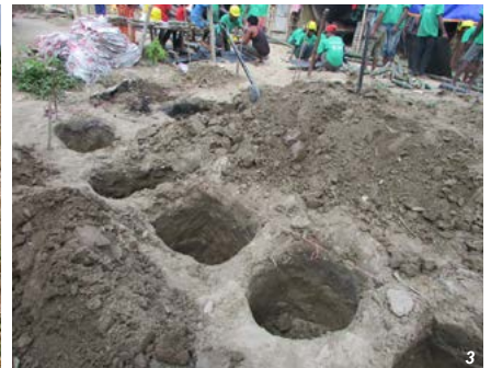
Left (1): Draw lines for foundation according to the dimensions and place the stakes in the ground. Check whether the stakes are at right angle using the 3-4-5 method. Centre and Right (2-3): Dig 21 post holes of 2' x 2' in the ground. (Photo credits: Habitat Nepal).
