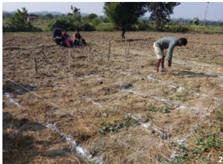
Left (1): Draw lines for foundation according to the dimensions and place the stakes in the ground. Check whether the stakes are at right angle using the 3-4-5 method. Centre and Right (2-3): Dig 21 post holes of 2' x 2' in the ground. (Photo credits: Habitat Nepal).
