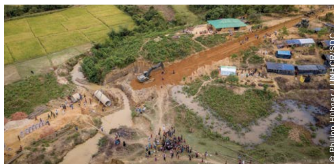
Major infrastructure (such as the Army road and culverts) was needed to convert a forest land into a liveable settlement.
