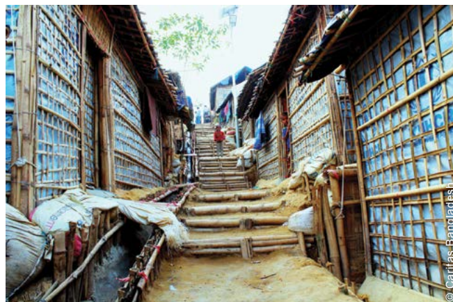
Shelter upgrades and localized site improvements (such as footpaths, stairs and drainage channels) were conducted in phase 2 to make living environments more adequate and protect households from the upcoming monsoon season.
