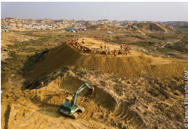
The Site Management Engineering Project was instrumental in conducting large earthworks to modify the challenging landscape.
