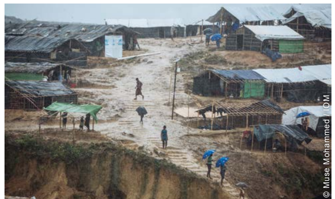
Access in and around the site was extremely challenging. When it rained, steps became impassable and perilous. Improved access became a priority in early 2018, in preparation for the monsoon rains.
