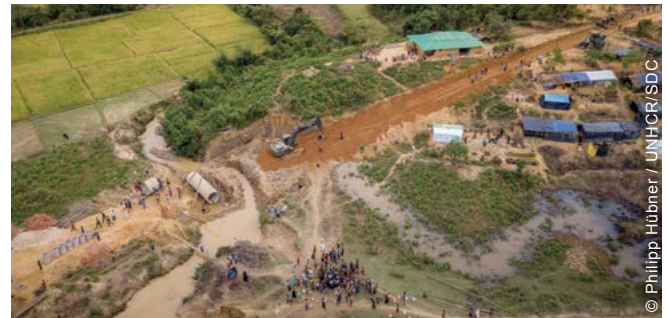
Major infrastructure (such as the Army road and culverts) was needed to convert a forest land into a liveable settlement.
