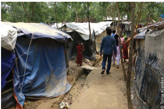
Makeshift shelters before the implementation of the upgrade phase of the shelter response were small, often fragile and highly vulnerable to weather hazards.
