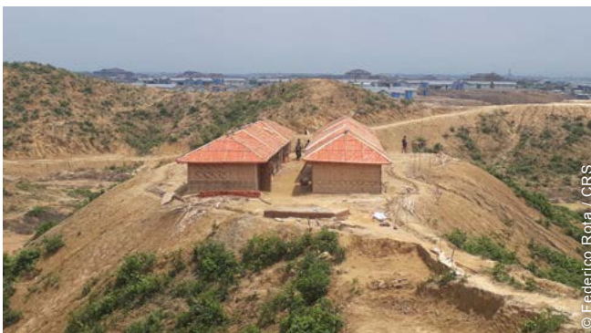
In the third phase of the response, Mid-Term Shelters were built on plots already prepared by site development partners.
