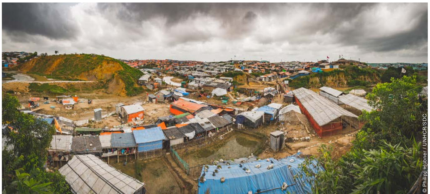
The site was completely transformed in just a few months. Less than a year before this picture was taken, this area was a natural reserve.
