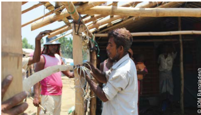
By involving refugees throughout the implementation, the project helped generating a sense of ownership over the shelters and their surrounding environment.
