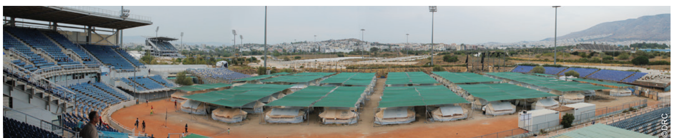
In Greece, many refugees were accommodated in tented camps. In summer, tents had to be shaded, also by building metal-framed structures (Elliniko, Athens).
