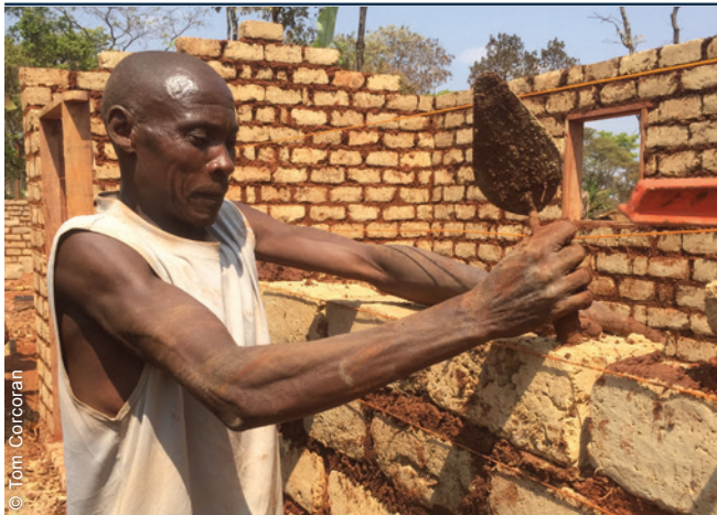
Mason laying the bricks of a shelter in Nduta refugee camp. Skilled builders from the refugee population were employed for the construction of the shelters.
