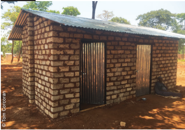
Duplex lime-stabilized shelter completed in Nduta refugee camp. Some of the shelters were designed to host two small families and followed the same design, but had two doors and a partition that divided the indoors in two units.
