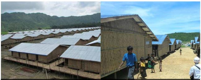
In some camps the shelters were raised from the ground and walkways constructed between the shelter. However, firewood was in such short supply that in some cases beneficiaries broke up the walkways for fuel. Rammed earth walkways had to be constructed instead.
