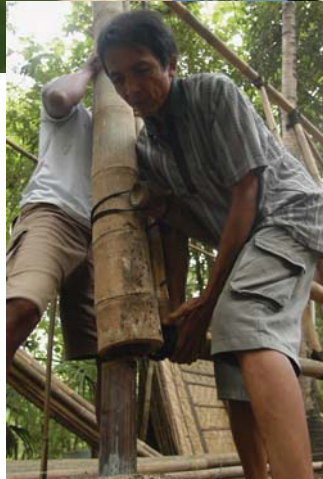
Connecting a vertical post to the foundation
