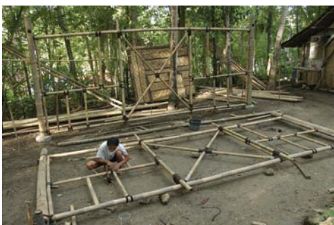
Prefabrication of a wall panel
