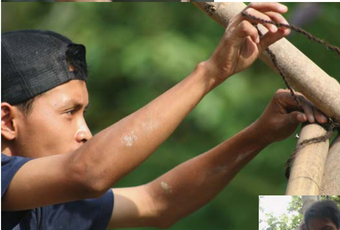
Bamboo being bound with string
