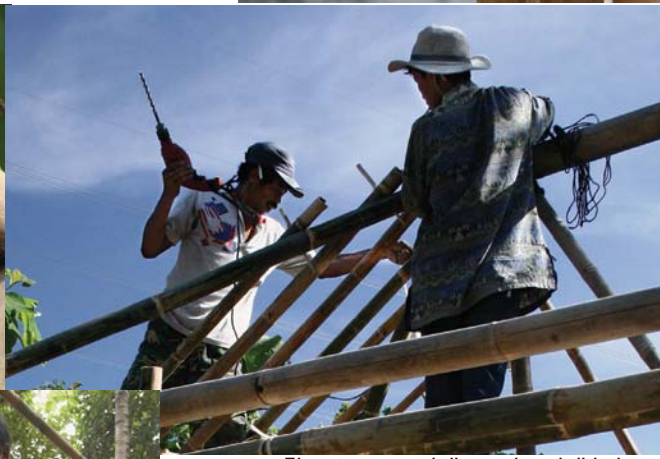
Electric power drills used to drill holes in the bamboo so that it can be pegged
