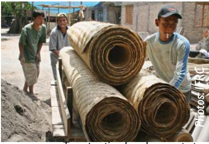
Transporting bamboo mats to a construction site
