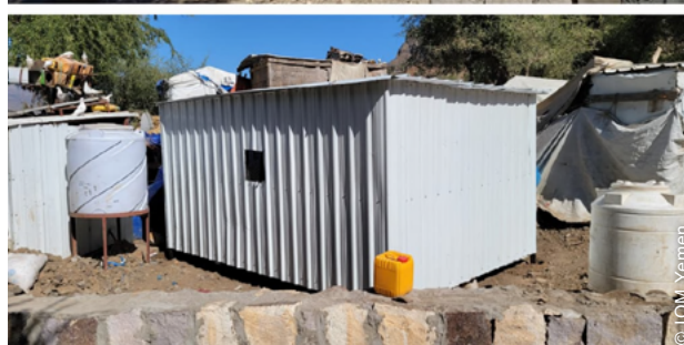
In some cases, the support was used to convert tents to metal sheet shelters.
