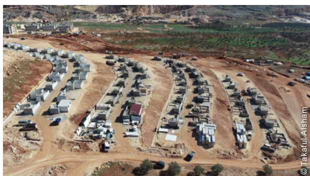
200 shelter units were installed following site planning and infrastructure works.
