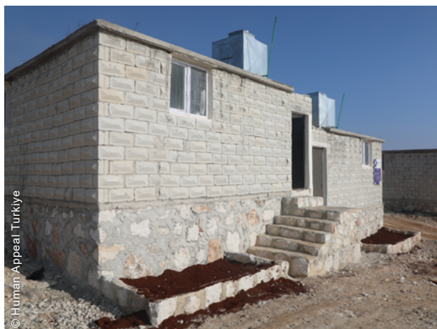
The project was implemented through contractors, while community participation was ensured by establishing site committees with various responsibilities.
