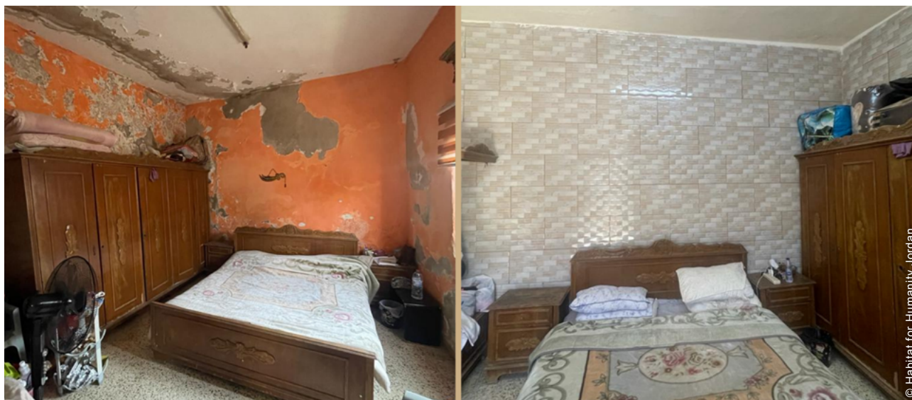
Upgrades such as damp-proof paint and tiling were installed to improve indoor living conditions. After initial challenges, the project shifted to a contractor approach.
