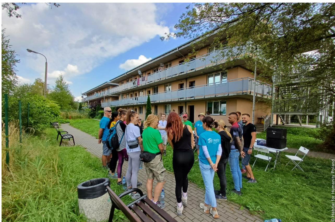
In the long-term phase, the project also renovated vacant buildings such as this one, which were then occupied through the Social Rental Programme. Volunteering played a key role throughout the project, both by participating in social cohesion initiatives and by actively contributing to upgrades and furnishing the apartments.
