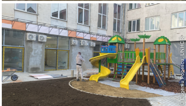
Selected public facilities were rehabilitated to provide multisectoral services to refugees and locals, alongside energy efficiency upgrades.
