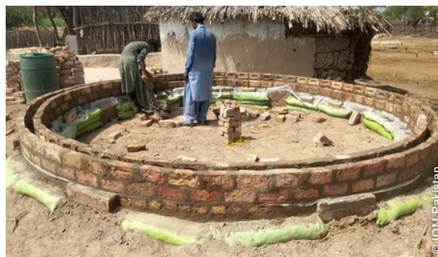
Pier foundations with sandbag infill were introduced following project extension.
