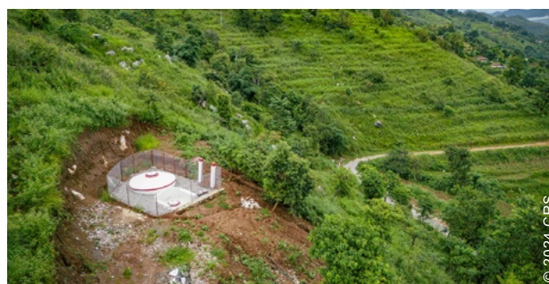
Beyond housing reconstruction, the project supported entire villages with the rehabilitation of water systems.
