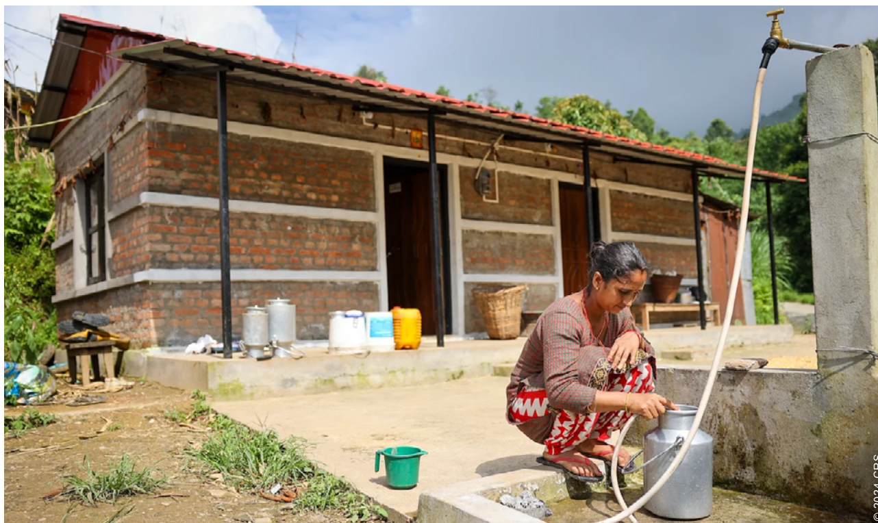
Targeted households were supported either with cash, in-kind materials or direct reconstruction for the most vulnerable cases.
