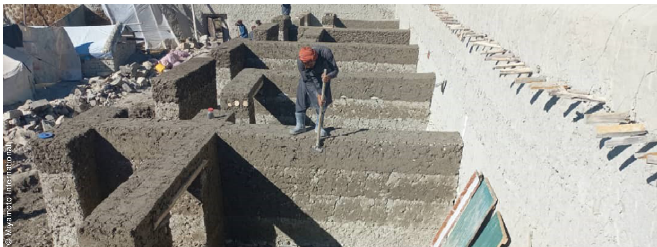
Focusing on connections, wall bonding and roof assemblies – where failures concentrated – yielded safety gains through modest, locally achievable enhancements.
