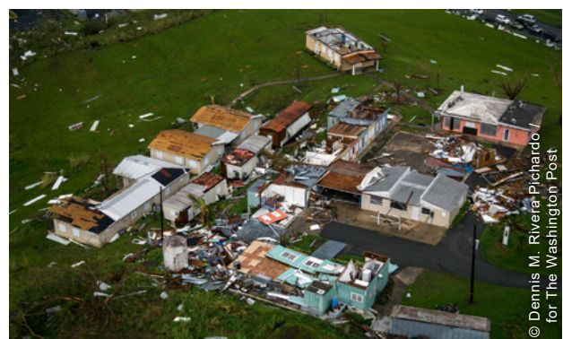
The hurricanes severely damaged roofs, walls and openings, and left the entire island without reliable electrical power for many months.
