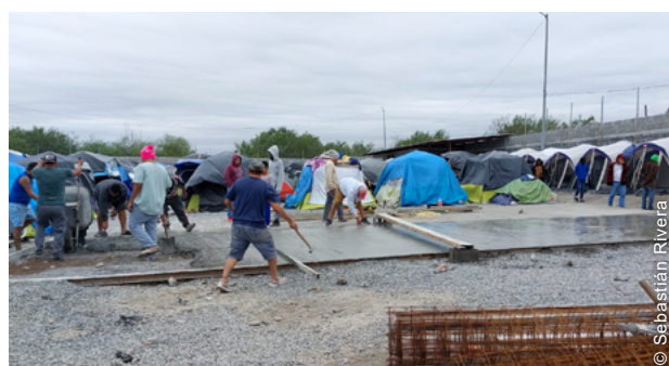
Largely implemented by the migrants themselves, the project used a phased approach, mostly because the site had been occupied before completion.
