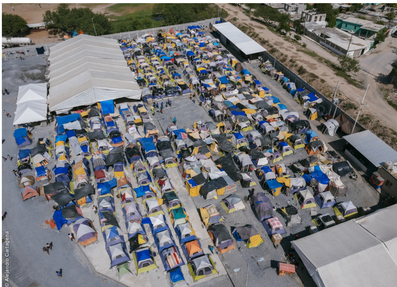
Beyond the family tents that were provided in the first phase, the project improved the general site infrastructure and included common areas and facilities.
