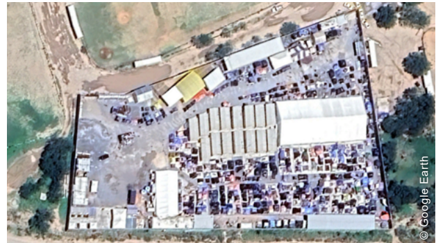
The photos show the site in the early stages of the centre (above, July 2022) and after the construction of the timber shelters (below, April 2023).
