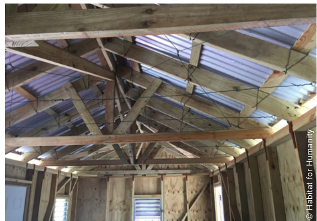
The project promoted safe practices for hurricane resilience through various means, including the construction of model houses also used for training.
