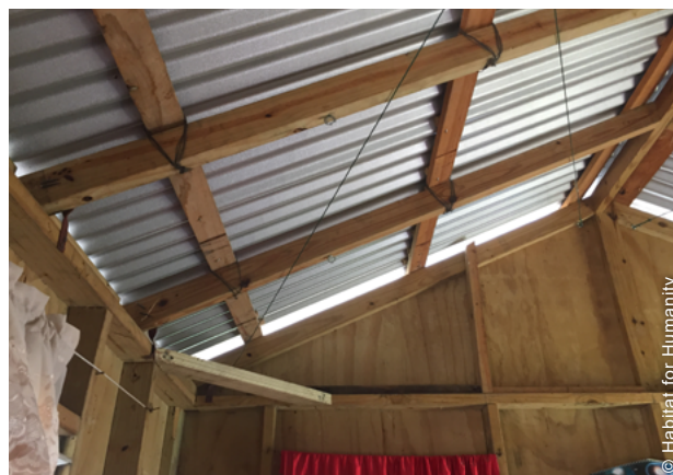
Galvanised wire was used to secure roofing elements and as cross bracing.
