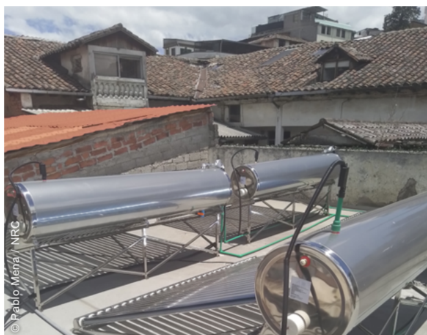
Solar panels were installed in some of the shelters, to reduce electrical bills.
