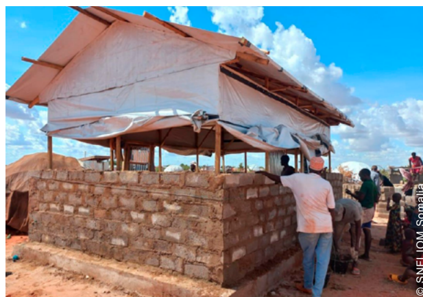
Upgradable walling materials, including concrete blocks and mudbricks, improve the durability and safety of Improved Emergency Shelters (IES)
