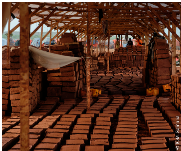
Earth-based construction, and primarily adobe (mudbricks), was promoted but could not always be adopted at scale due to limited familiarity of the techniques and perception barriers.
