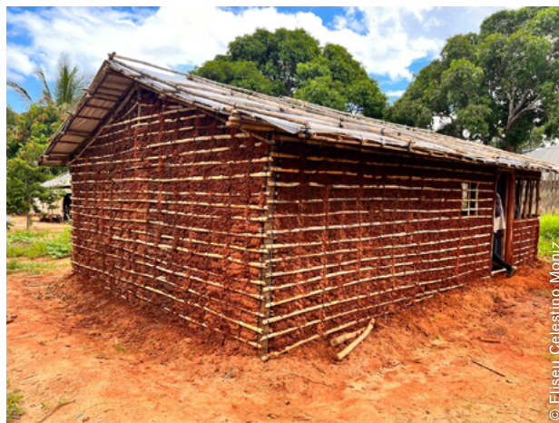
The shelters provided by the project incorporated local knowledge and traditional techniques and materials.
