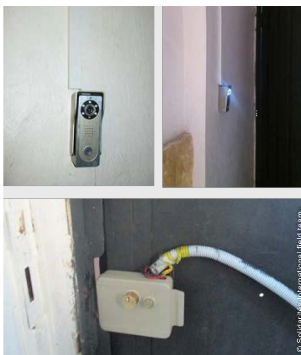
Video phones were installed for people with limited or no mobility, allowing them to monitor their visitors and control the entrance door remotely.
