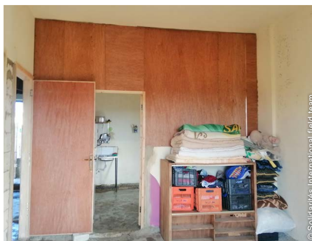
Partitions were installed to separate the kitchen from the living/sleeping space. This improved hygiene and allowed more privacy.
