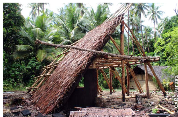
Model house structures were built at the community level on Maewo, to demonstrate traditional safe construction principles for all shelter training and awareness activities.
