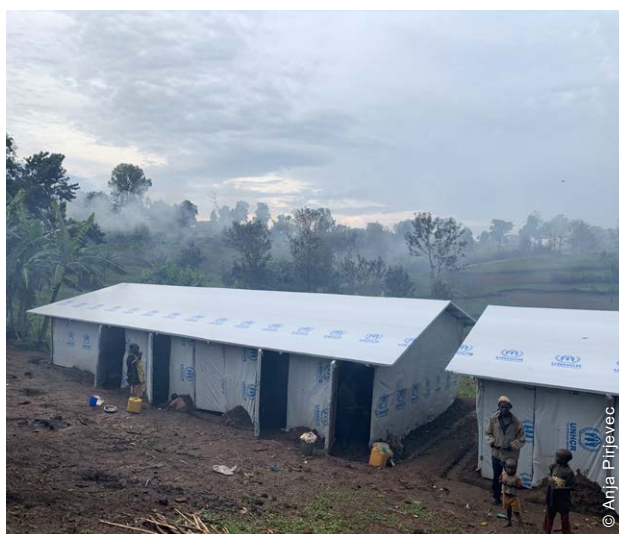
79 collective shelters were built in host communities to support IDPs sleeping in the open air or in public buildings. Collective shelters were partitioned with separate units for eight households.
