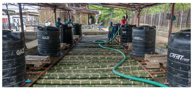
The orthoboric solution used for the treatment of bamboo was selected for its ease in processing and its non-toxic nature.
