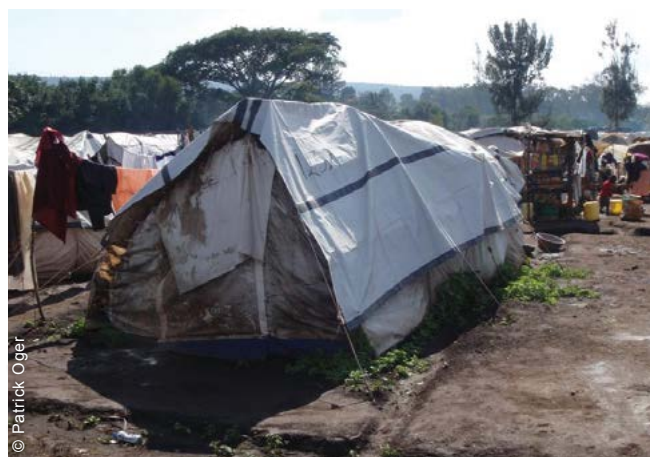
A good-quality tarpaulin can resist up to a year or longer. It can be used for multiple purposes, such as covering older plastic sheets to provide waterproofing.
