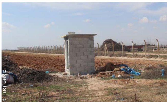
The project also provided rehabilitation of water supply and sanitation facilities.
