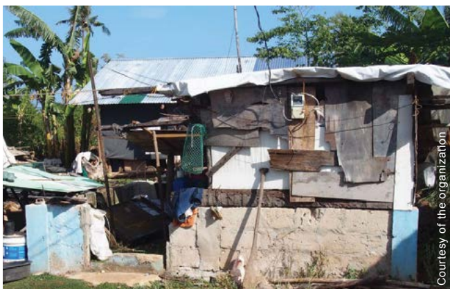
A year and a half after the typhoon, many houses were in very poor structural conditions. For this reason, repair and retrofitting assistance was not an option, although this would have reached more people because of the lower costs.
