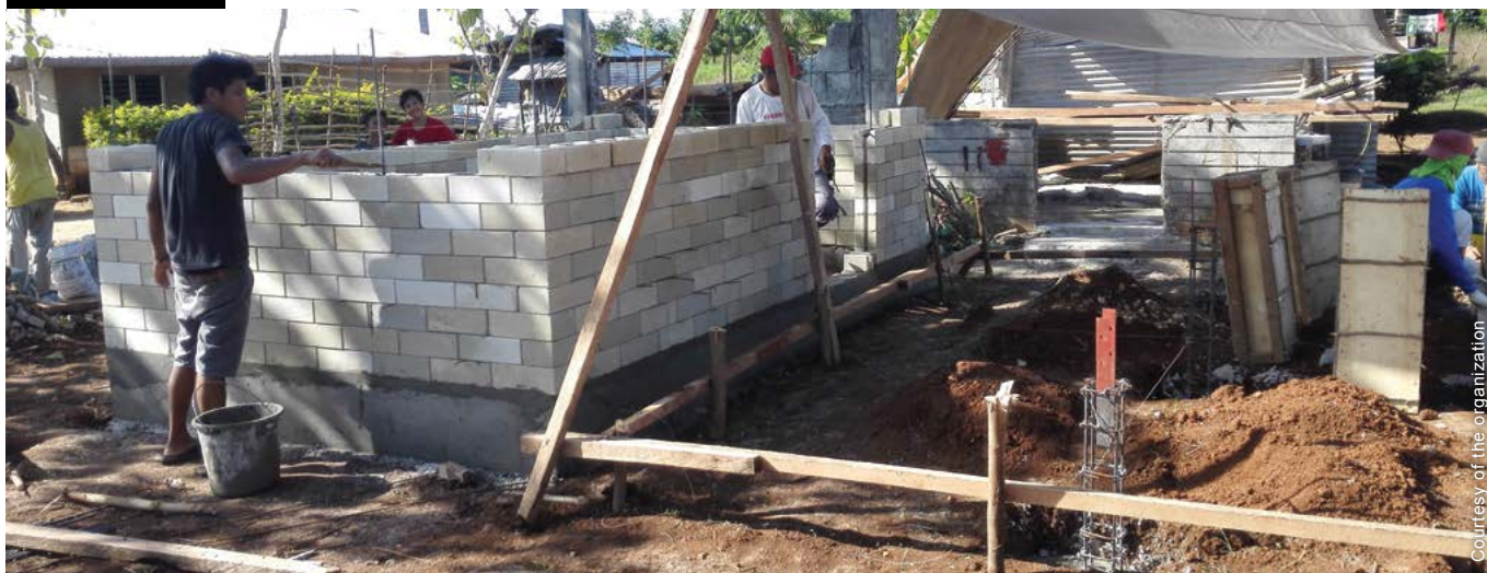
The construction was owner-driven and implemented via conditional cash transfers. People could choose between a full-timber house or a hybrid ICEB-timber structure.
