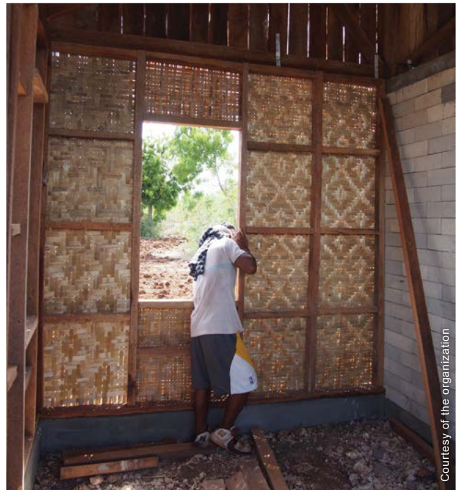
The adjoining room was made with a structure in coco lumber protected with a termite treatment, and an amakan walling. This could be replaced or re-design, so some families could built extensions for small kitchens and dining areas.
