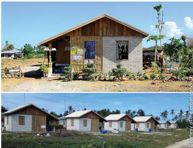
Core houses were built to resist typhoons and earthquakes and have an expected lifespan of 20 years for the core and 10 for the extension.
