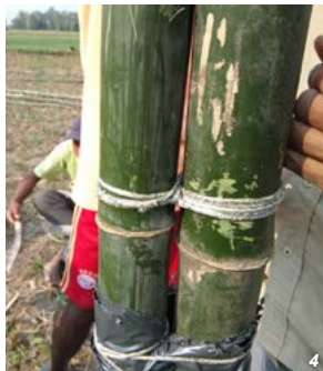
Left (4-5): Cut the required length of floor and roof posts with saw, tie them together and wrap them with polythene sheet. Cut the upper ends of the posts with a fish-mouth cut. Right (6-7): Place and tie floor beams to the bamboo floor post with rope. Place the next set of beams on top, perpendicular to the beam below. Place split bamboo joists above the floor beams. (Photo credits: Habitat Nepal).
