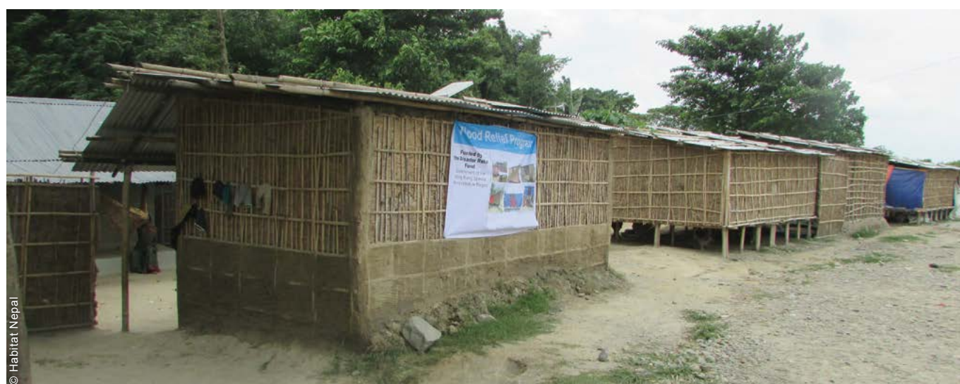
Shelters included mitigation features, such as raised floors, bracing and secure connections, and allowed for some adaptations, such as the upgrade of floors and walls.
