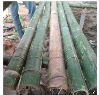
Left (4-5): Cut the required length of floor and roof posts with saw, tie them together and wrap them with polythene sheet. Cut the upper ends of the posts with a fish-mouth cut. Right (6-7): Place and tie floor beams to the bamboo floor post with rope. Place the next set of beams on top, perpendicular to the beam below. Place split bamboo joists above the floor beams. (Photo credits: Habitat Nepal).
