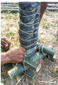
Left (8-9): Tie bamboo posts to the anchorage and place it inside the post hole. Then fill the hole with debris and tamp using wooden tamper. Right (10): Tie diagonal bracings of required dimensions to the roof post. Then tie the horizontal bracing at lintel level. Place the roof beams on top of the bamboo post and tie with rope. Place the cross bracings at roof level and then tie to the beams with rope. Right (11): Place bamboo purlins on top of the roof beam and tie with rope. Arrange 8 CGI sheets over them leaving one sheet width vacant in the middle. Tie 2 layers of purlins together to hold the CGI sheets in place. Place the remaining CGI sheet over the void and place 3' length purlins on top of each purlins below to hold the sheet down. This provides air movement inside the shelter through the roof. (Photo credits: Habitat Nepal).
