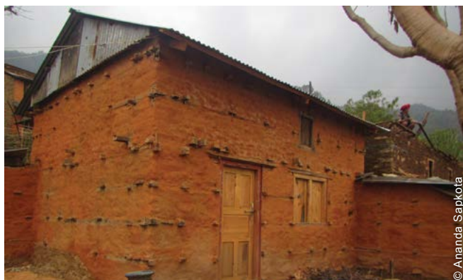
Designs were flexible and allowed the use of local materials without compromising on compliance with the building code.
