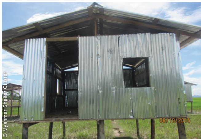
Contractor-driven approaches were tried and later rejected by IDPs and the Shelter Cluster (Nidin IDP Camp, Kyauk tau Township).
