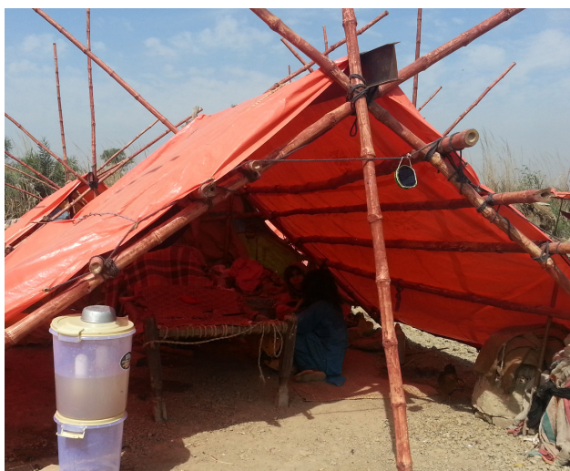
An example of an emergency roofing kit which will later be used for a transitional shelter then again for the roofing elements of a permanent flood resistant shelter.
