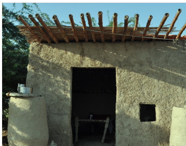
The second, transitional stage in the life of a roofing kit. This temporary hut, lived in for about a year, will be dismantled and the roof will be used for a permanent house. This saves around US$ 111 from the cost of the new shelter.
