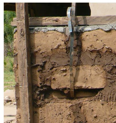
Fixing the roof to the wall: a wood block has to be placed between the mud bricks and strapping to stop it tearing through the wall. Photo: CRATERre
