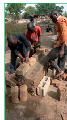
Barrier against water uprising : cement mortar (350kg/m 3 )
