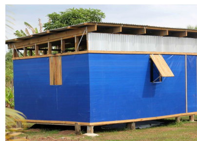
No rigid wall linings were permitted, so plastic sheeting was used instead.
