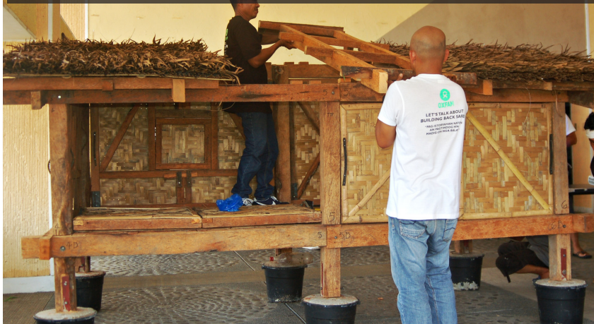
Demonstration of prototype collapsible transitional shelter. While the design is in development, beneficiaries are assisted through the standard voucher modality. Photo: Oxfam.
