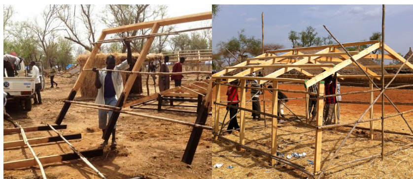
Posts were treated with engine oil before being dug into the ground. The community was responsible for the final erection of the shelters. Photos: UNHCR
