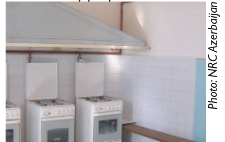
Kitchens before and after upgrade
