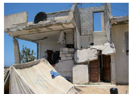
A blockade on construction materials prevented houses from being built. Photo credits: CHF
