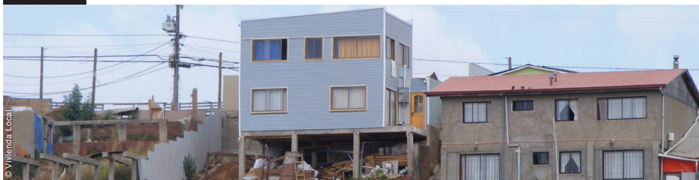
Architects and local NGOs helped affected people rebuild their damaged houses, thanks to the “assisted self-construction” subsidies provided by the government.
