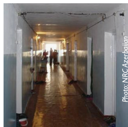
Corridors before and after upgrade
