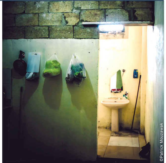
Bathrooms were also repaired and upgraded under the project.
