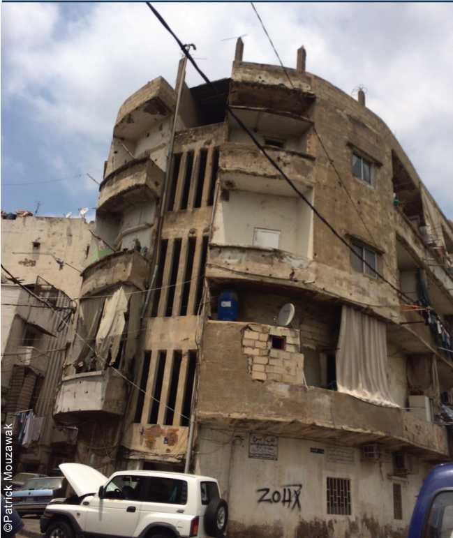
The project made basic upgrades, but it became challenging to find enough buildings in the targeted communities.
