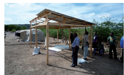
Prototype transitional shelter Photo: Joseph Ashmore
