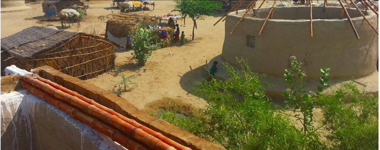
Two different types of shelter: in the foreground, an unfinished, square, flat-roof house with compound bamboo ring beam on top of the walls. To the right, a round house (known locally known as "chulla"). This was the first time people in this village had constructed permanent shelters. Photo: Magnus Wolfe Murray
