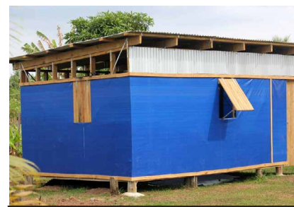
No rigid wall linings were permitted, so plastic sheeting was used instead. Photo: Habitat for Humanity Fiji
