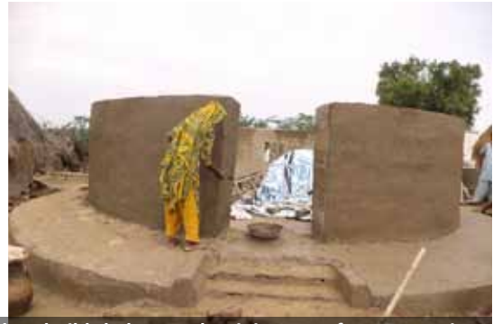
Women plastering their one room shelters. The project provided cash to build shelters and training on safer construction with incremental improvements such as stronger plinths and footings to walls. Households chose their own shelter design.
