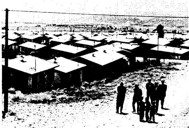
Prefabricated housing built by the Turkish Government at Lice following the earthquake of September 1975. Many families objected to the form and siting of the housing. These objections related to their lack of participation in what was provided, and the cultural and climatic unsuitability of the housing.
