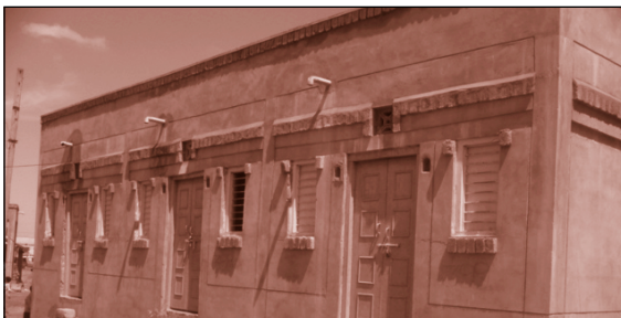
Contractor-built houses in Gujarat
